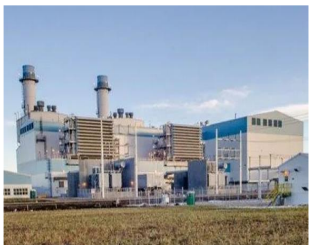
Shepard Energy CO 2 Capture Plant in Calgary, AB utilizing Delta technology
