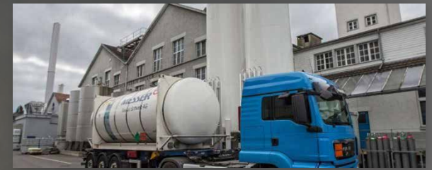
ASCO Carbon Capture Plant, Switzerland
