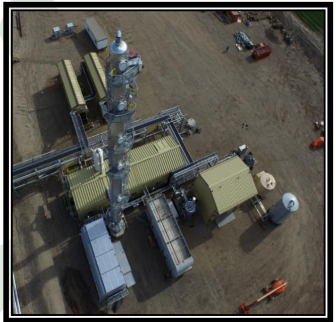
Delta's modular LCDesign CO 2 capture system.
